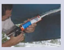
This high-performance polyurethane adhesive sealant becomes tack-free in 24-48 hours, and completely cures in 5-7 days with no shrinking. The seal is extremely strong, retaining its strength above or below the waterline. Stays flexible-allows for structural movement. Stress caused by shock, vibration, swelling or shrinking is effectively absorbed. Has excellent resistance to weathering and salt water. Check the bonding and sealing jobs this product can handle for you:
