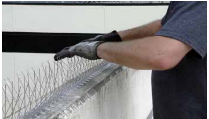
Stainless steel spike installed on rooftop parapet wall.
