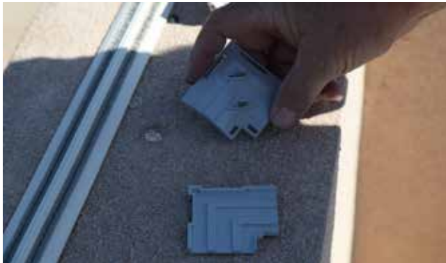
Product Installed: Bird Jolt Flat Track®
