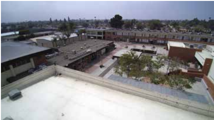
High school rooftop installation area.
