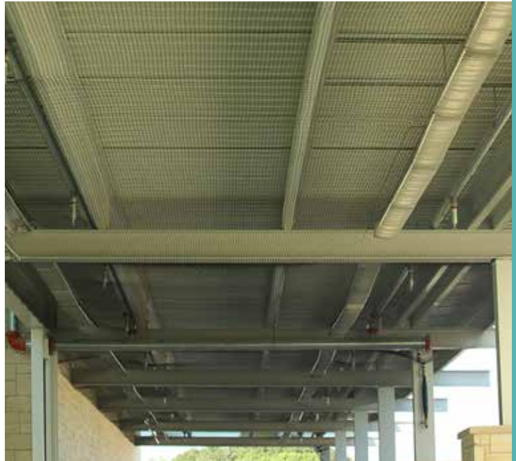
Completed installation of Bird Net 2000 Heavy-Duty Netting™.
