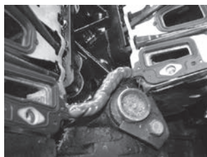
PermaDryPlus® intake gaskets installed dry: RTV used for end seals.
