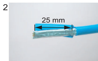
2 Remove the outer sheath by approx 25 mm. Be careful not to damage inner shield and cores.
