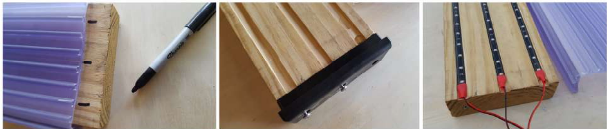
FIG 4 Marking, Planning and cutting grooves for LED strips
