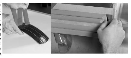
Once fully attached, use the burnishing tool to apply additional pressure to the entire PontoonGuard, ensuring the pressure sensitive adhesive is firmly attached.
