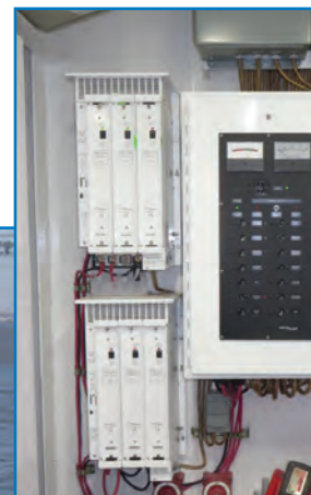
Engine room installation.
