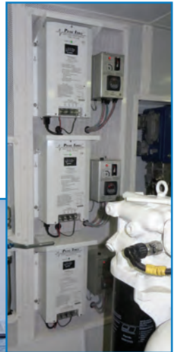
Installation with optional PT-MCU Control/Monitor
