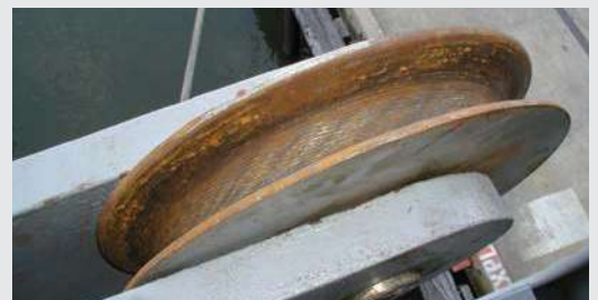
Contact with rusted, uneven surfaces will shorten the service life of synthetic lines due to abrasion and cutting damage.
