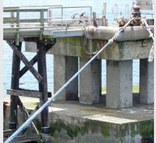
Mooring lines with twist induced.
