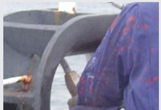
Coating removal using a needle scaler
