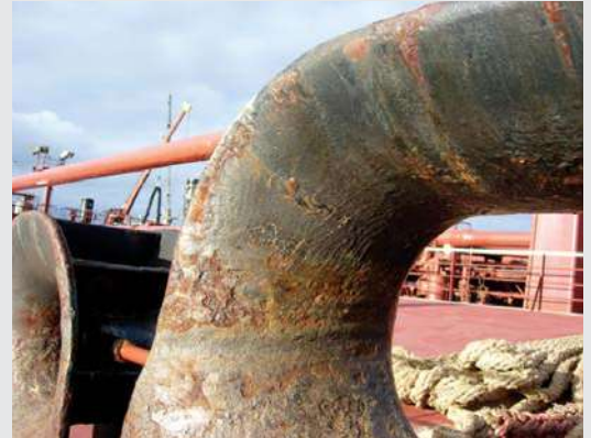
Rust damaged chock typical of crude tankers.
