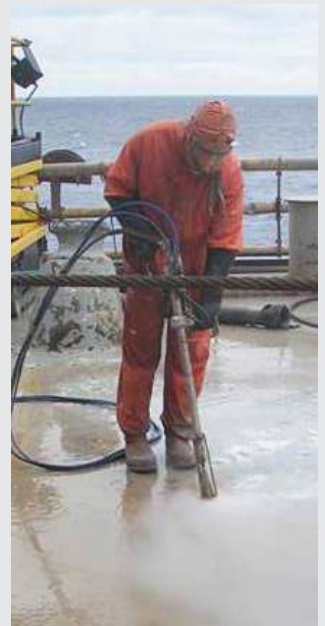
International standards are applicable to surfaces produced by a range of hydroblasting equipment, providing it is capable of cleaning to the visual standard depicted.
