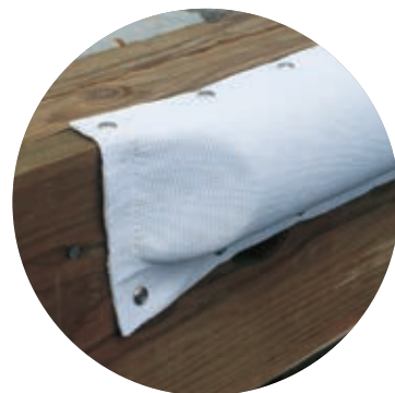
"Top-of-Dock" installation method
