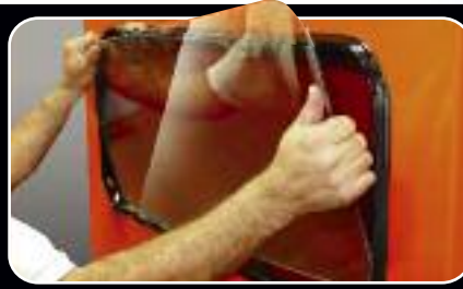
2. Lubricate Locking Gasket. Then slide glass in bottom first.
